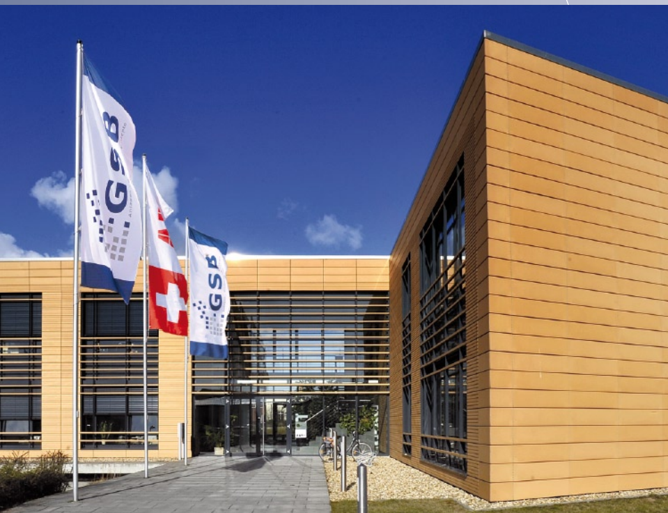
GSB administration and production facility, Rommerskirchen
