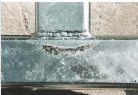
Burned oil during welding
